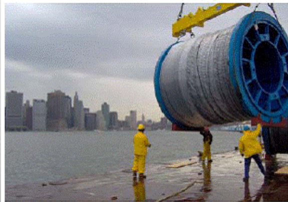
Cable reel off-loading, September 2006
