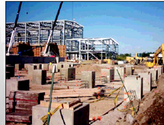
Long Island converter station under construction, August 2006
